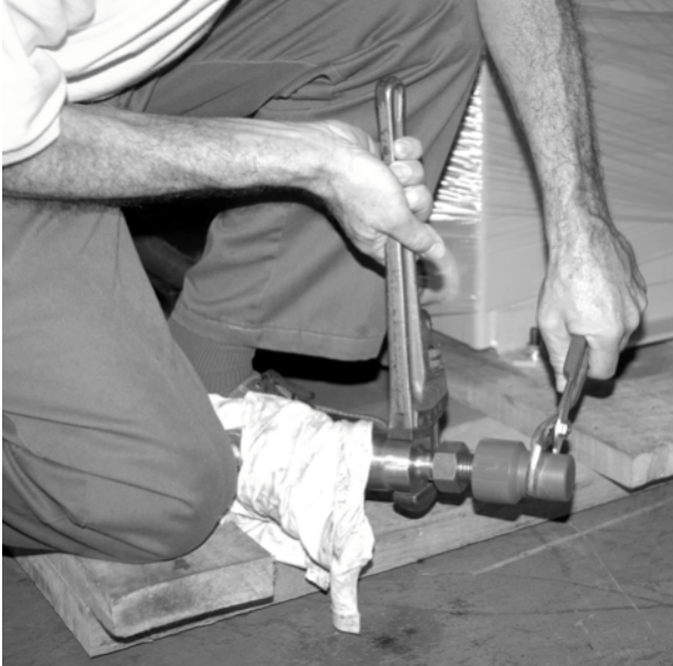
Figure 6: Attach the UHMW base for the rod to the switch operation rod
